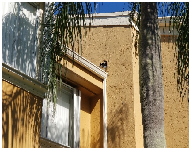
Photograph 12: Opening in the exterior wall
