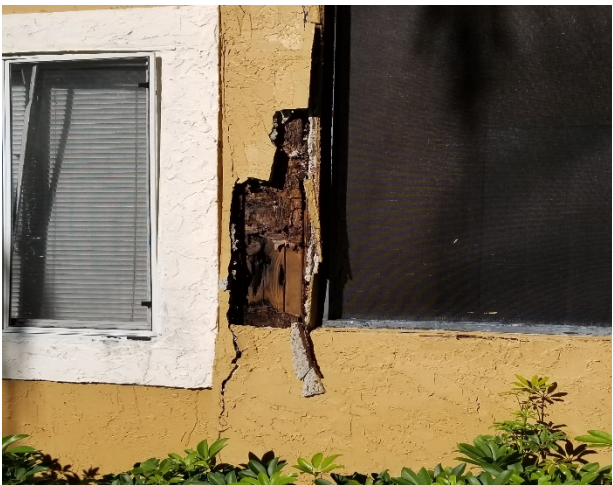
Photograph 11: Opening in the exterior wall
